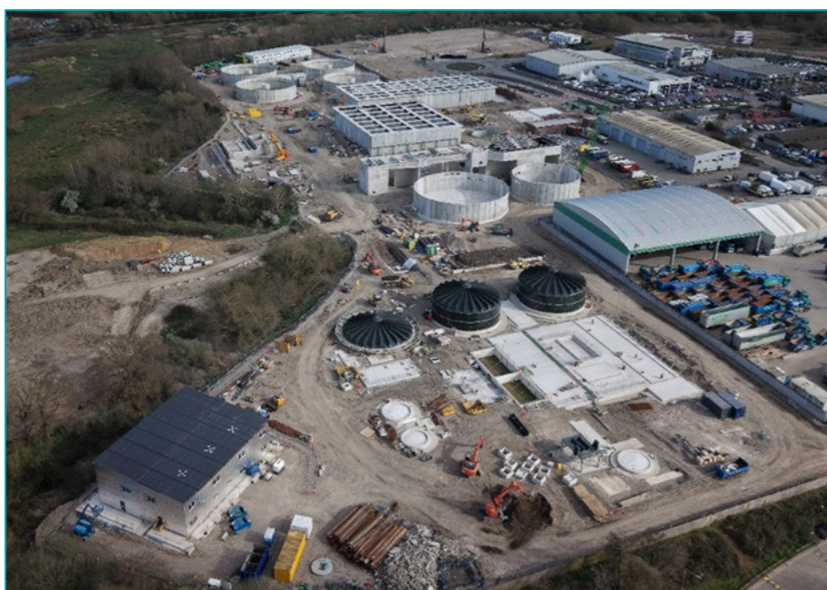
Figure 9: A new sewage treatment works is being developed as part of the Weyside Urban Village project. Source: Thames water
