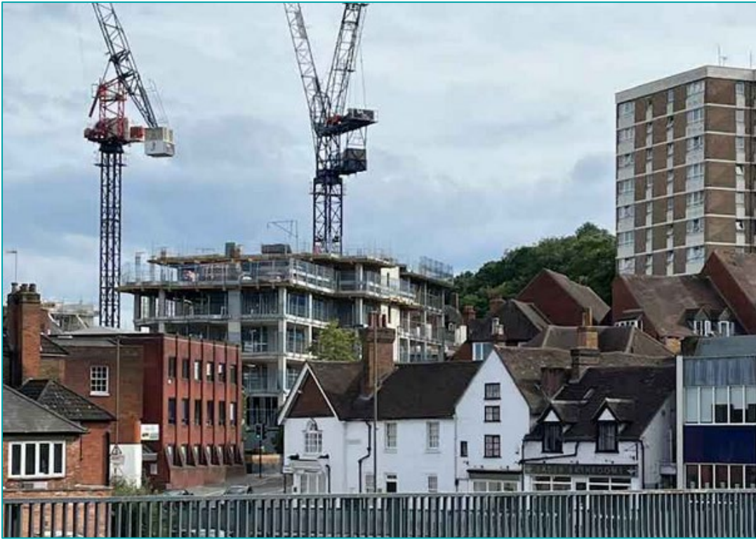
Figure 6: Guildford Plaza (student accommodation) during construction
