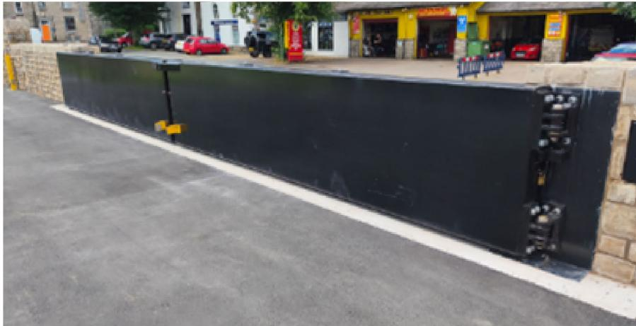
Here is an example of a hinged single leaf flood gate which is open. As you can see it rests flat against the wall when opened, allowing pedestrian access.
