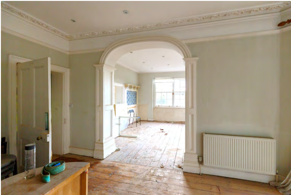
Existing arched opening to be infilled
