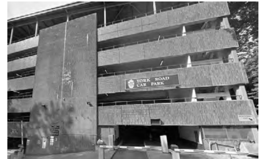
York Road Car Park
