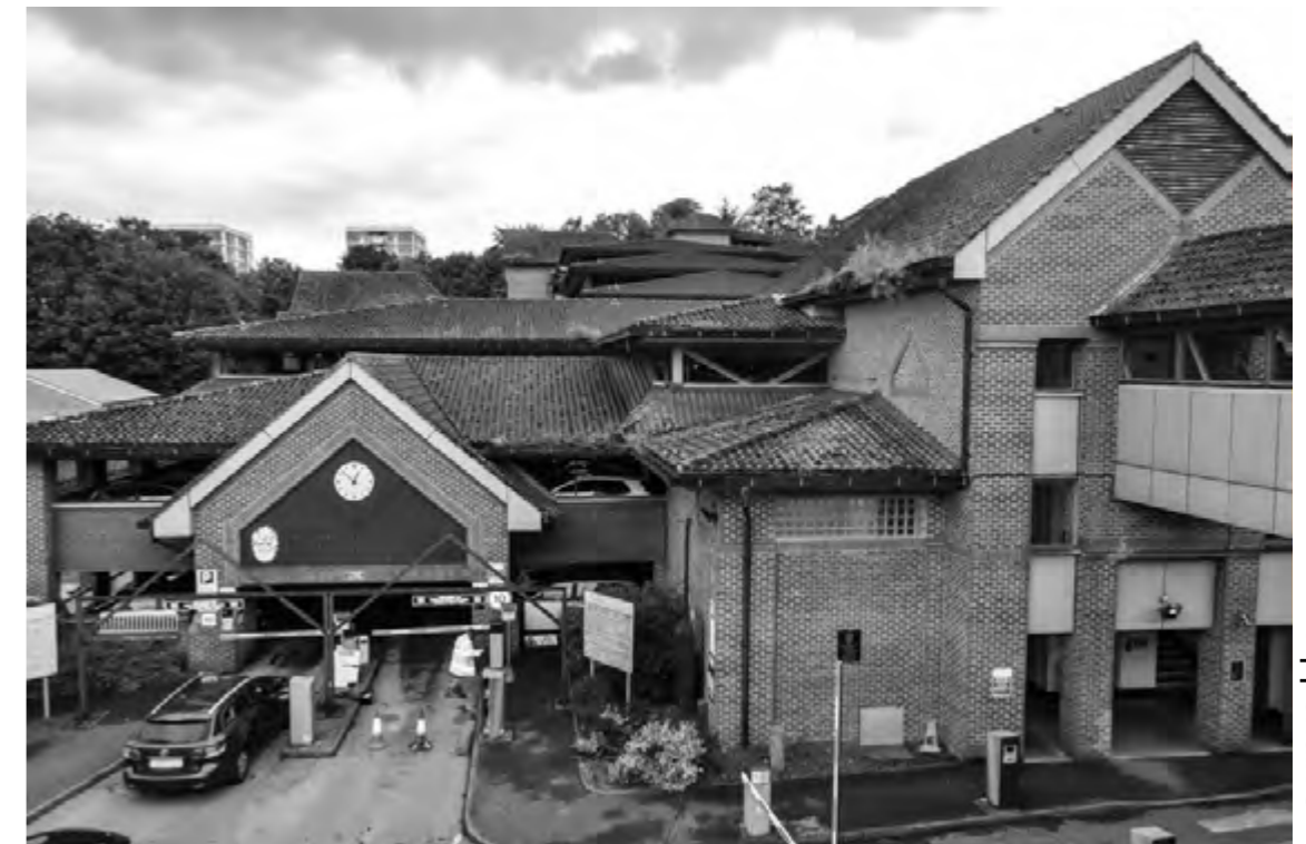
Farnham Road Car Park
