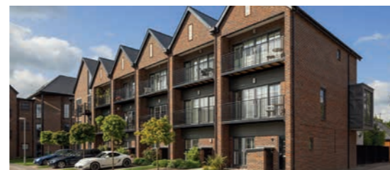
Gable fronted warehouse style brick buildings that celebrate the Pump House
