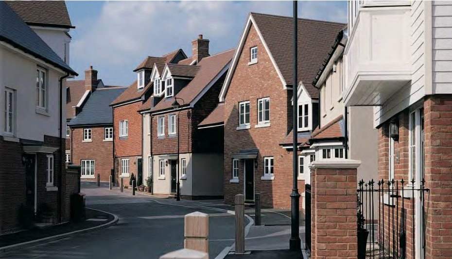
Ingress Park, Dartford (GSA)
