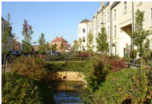
Formal swales incorporated within an urban context, drawing green infrastructure into the streetscape.
