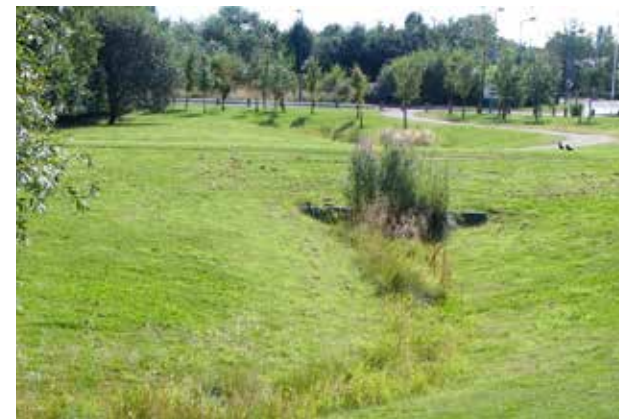
Where attenuation areas are mainly dry, other than in storm events, they can be used as open space.
