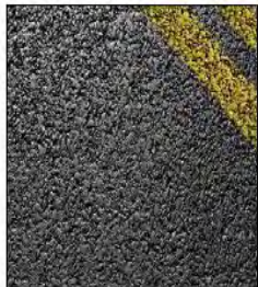
Bitumen Macadam Road Surface or Similar
