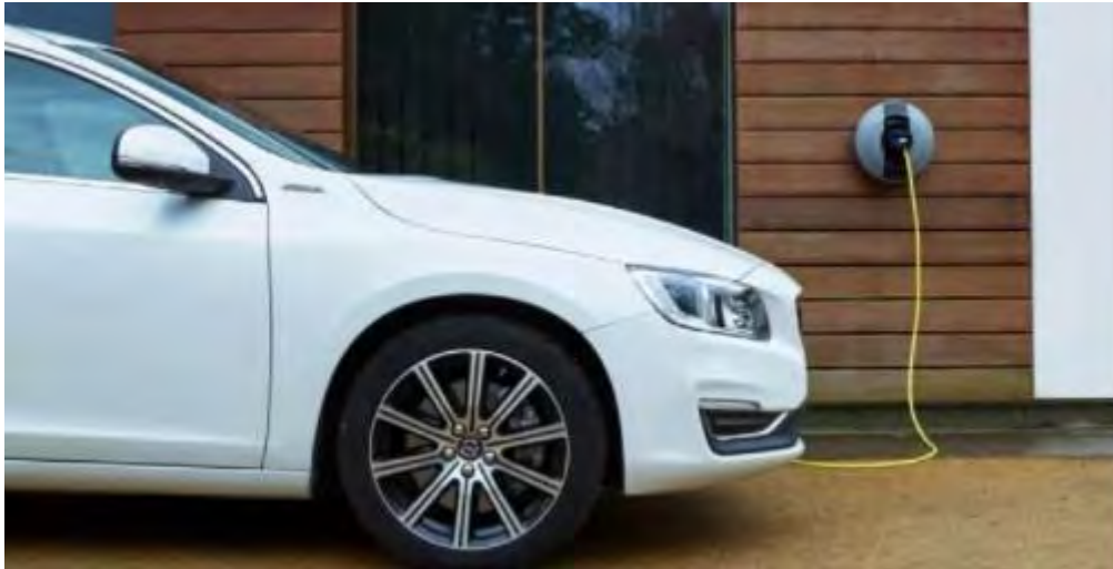
Figure 8. Residential charging point
