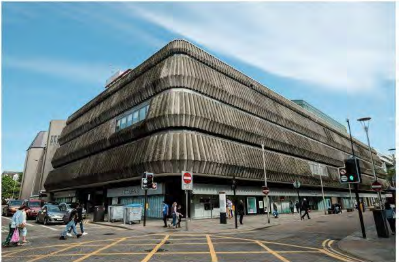
Norco House, the former John Lewis, Aberdeen – Covell, Matthews & Partners (1966-70)
