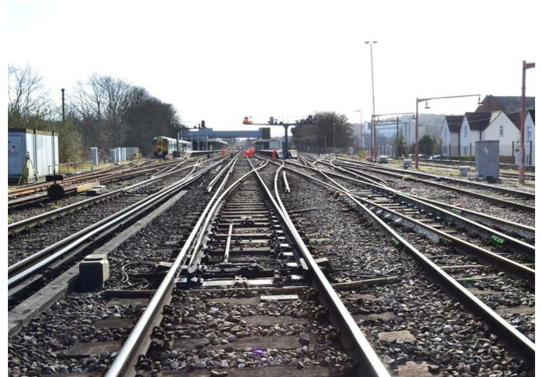
Engineering work during Redhill platform 0 construction , Arup
