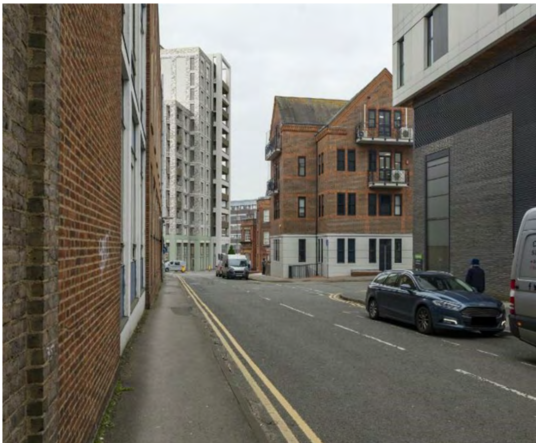
Note the North Street Site has been rendered in CGI not as a wireframe .
